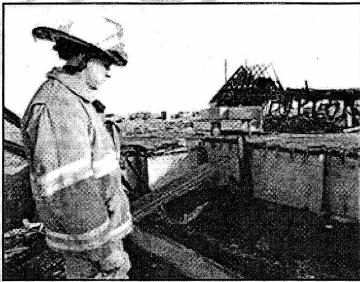
A firefighter surveys damage to a luxury mansion in Boulder, Colorado.
