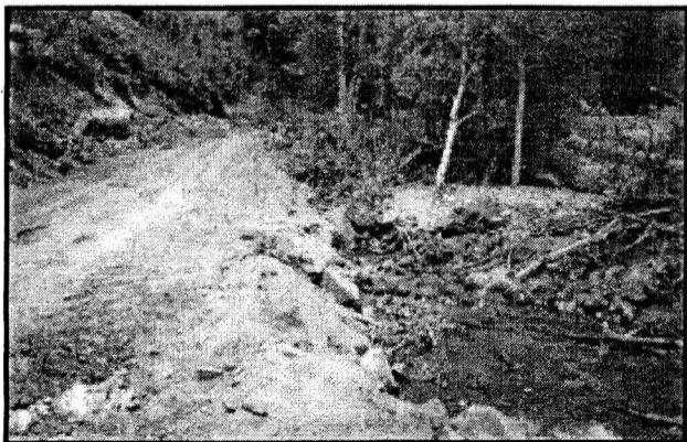
The rebuilt road collapsing into the Jarbridge River.
