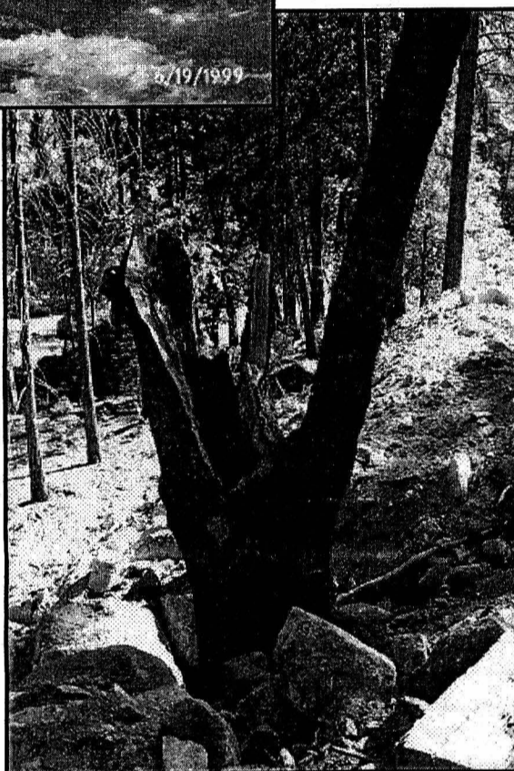
This is how they "save" ancient black oaks and the bat that roosts in them. This well is supposed to be dug around the base to "save" the tree from the fill which has been dumped on the formerly rich habitat slope. A sad joke which would not save the tree in any case. The tree which was marked to be saved has been bashed to smithereens by heavy equipment.
