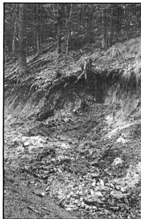
A slump on Jack Road at Cove/Mallard
