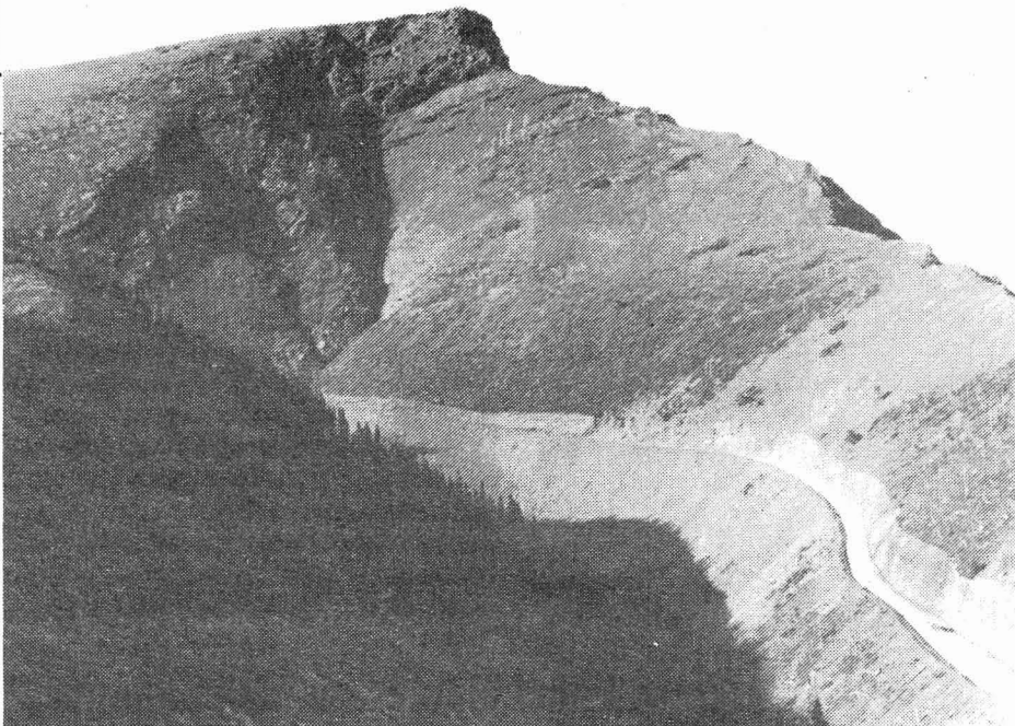
Bighorn Sheep summer, fall and winter range. The road was built right along a former sheep trail. The valley was also prime Grizzly Bear habitat. Most of the road was cut through bed rock. It can never be reclaimed.
